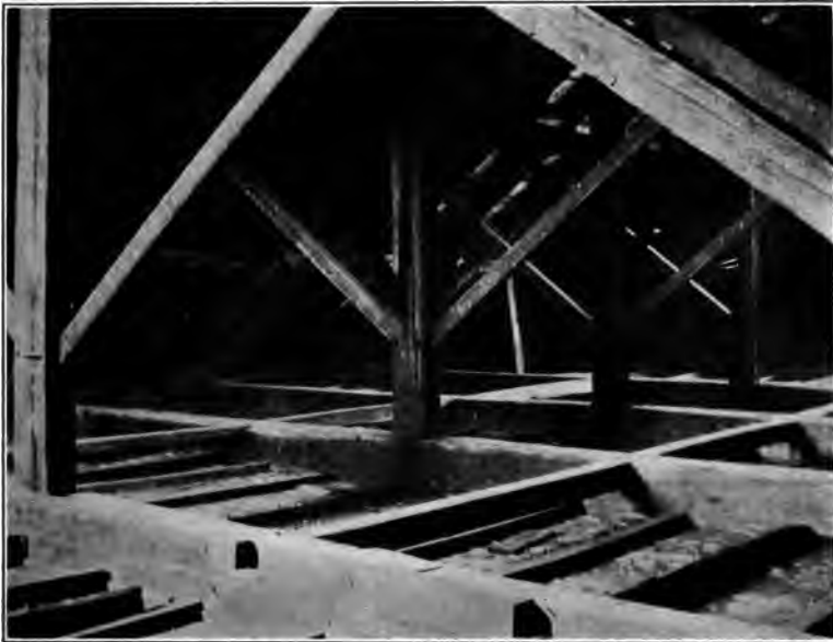
HEAVY ROOF TIMBERS IN THE ATTIC OF THE MEETING HOUSE
